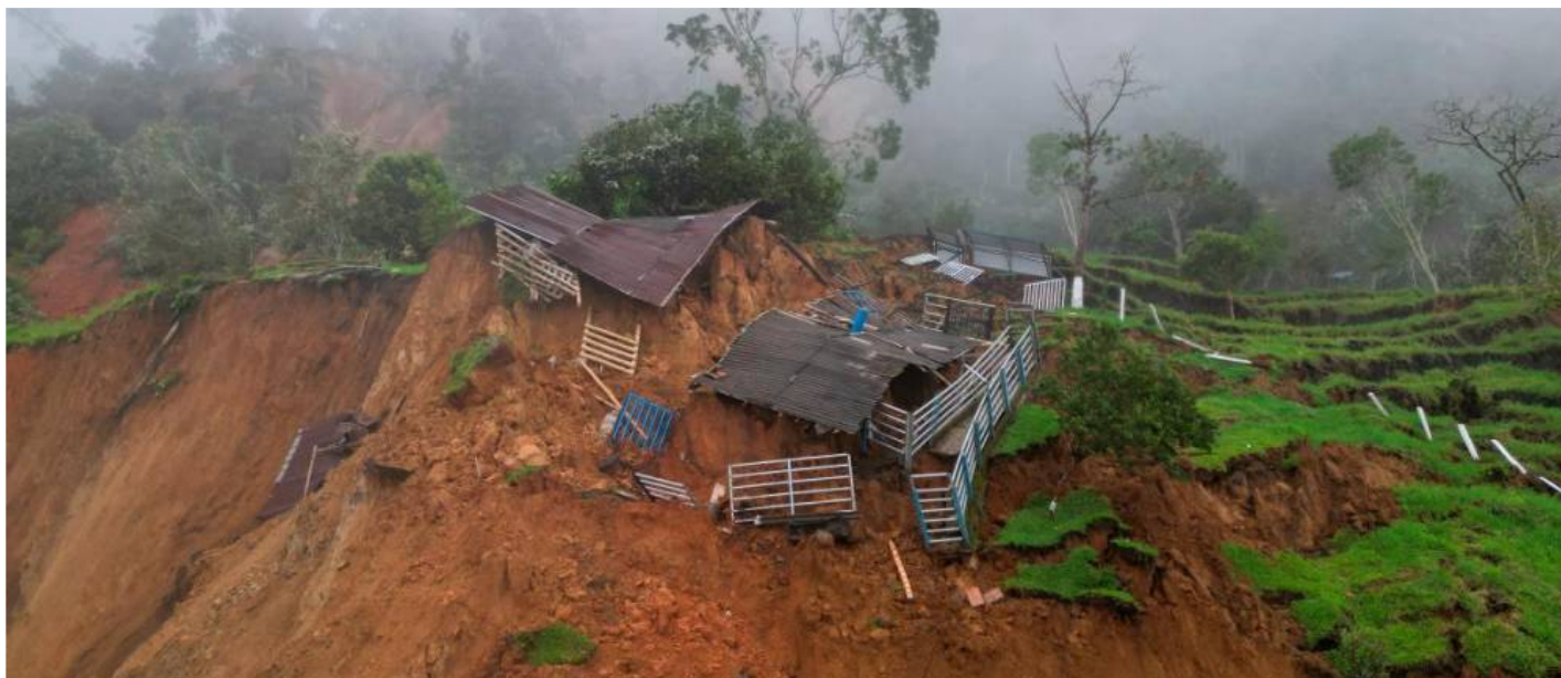
Landslides caused by heavy rains in Rosas, Cauca. December 2022. Source: El Universal.
