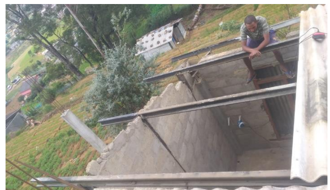
An SLRCS volunteer replacing and repairing the roof of a damaged house in Kandy district (Photo: SLRCS)
