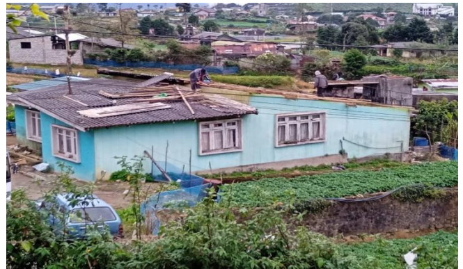
SLRCS volunteers repairing roofs of damaged houses in Nuwara Eliya district (Photo: SLRCS)
