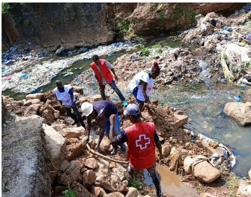
Volunteers supporting community drainage cleaning
