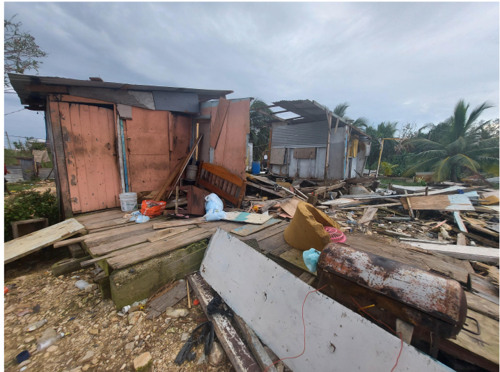
Destroyed homes after Hurricane Lisa, Belama
