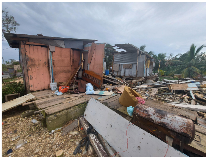
Destroyed homes after Hurricane Lisa, Belama
