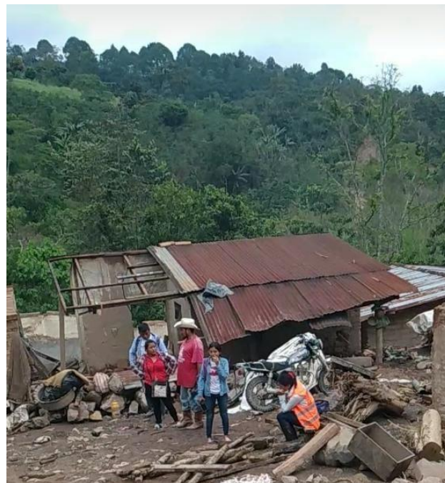
Damage assessment of destroyed houses in the community of Platanares, October 2022. Source: Cabañas CODEM, Copán.
