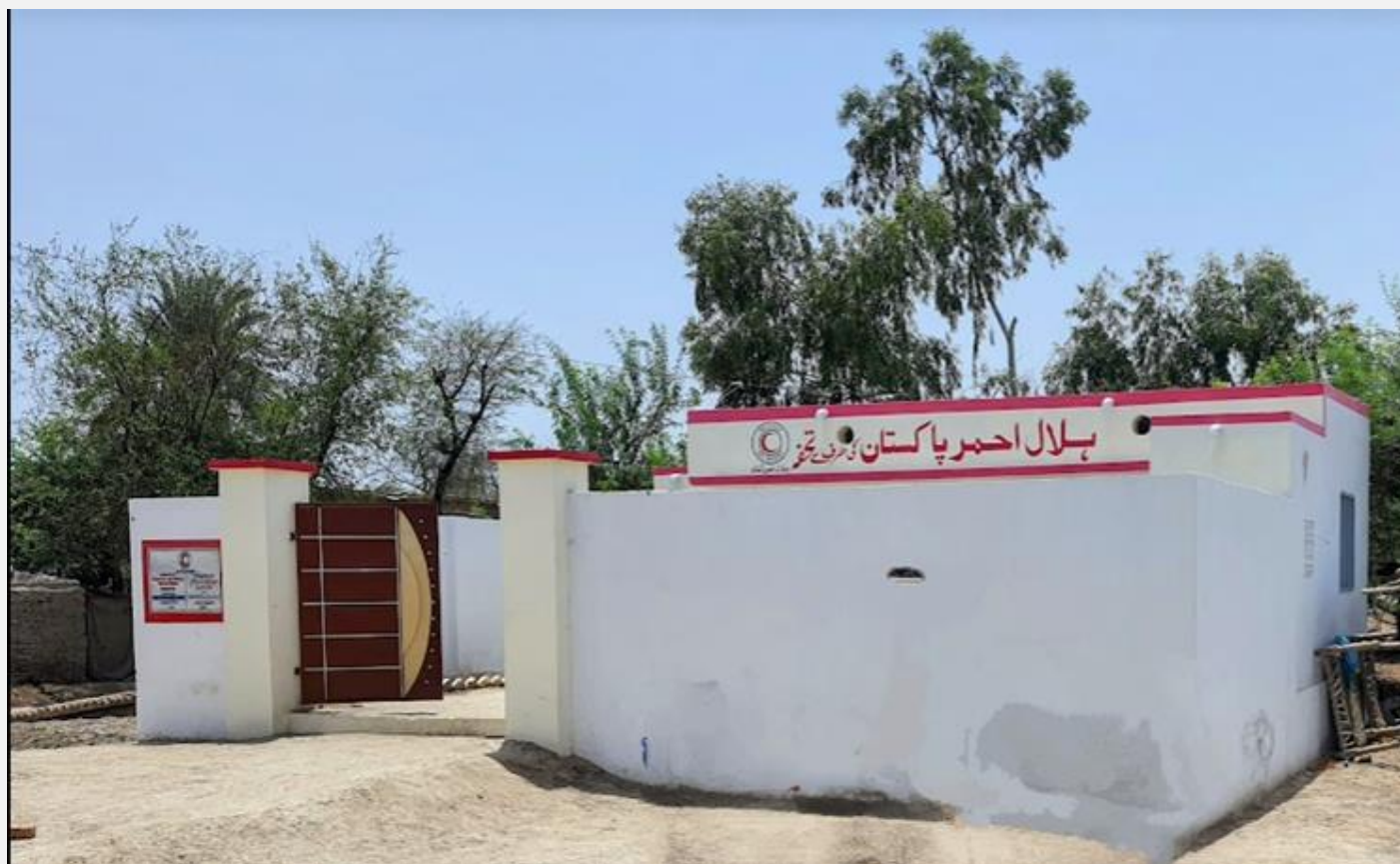
A model house constructed by PRCS with technical and financial support from IFRC in Larkana district. Some 40 model houses will be constructed under the Floods Recovery Programme across Pakistan and will be given to the most vulnerable communities affected by 2022 monsoon floods. (Photo: PRCS)
