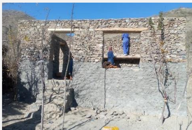
Shelter repairing in Tani Khail village of Spera. district (Photo: IFRC)
