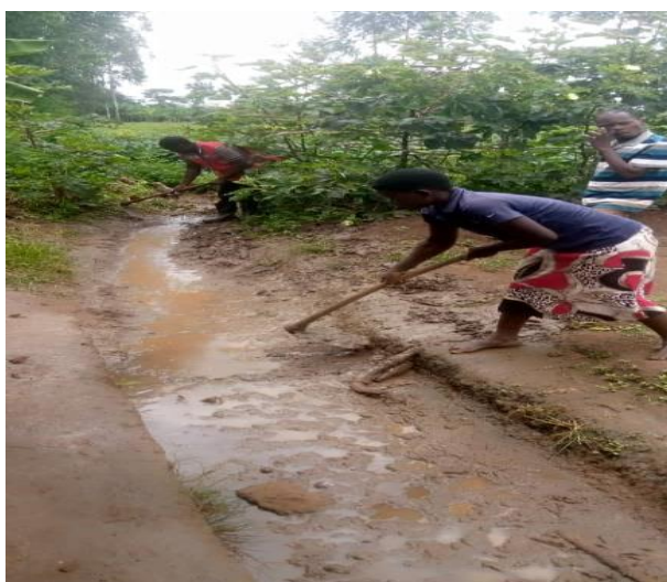
Figure 3: Volunteer directing the community members in digging trenches in Simu subcounty, Simu corner village, Bulambuli
