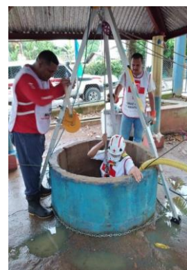
Cleaning of wells in the municipality of El Rama, October 2022. Source: NRC.
