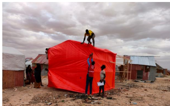
SRCS Volunteers and participants from the beneficiaries are supporting each other in the erection process of the emergency shelter
