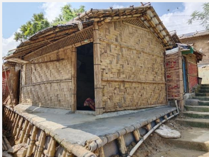
Mid-term shelters in camps 11 and 12 were constructed along with site development works, such as stair, protection wall. (Photo: IFRC)
