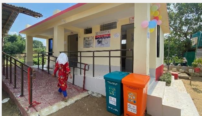
A WASH block at an academic institute (school) is conveniently used by its students. (Photo: IFRC)
