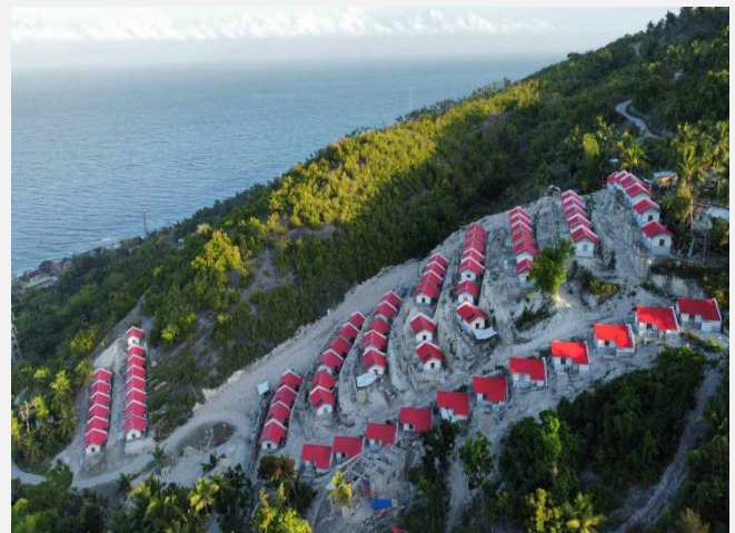
Another glimpse of the Full Shelter Assistance project in Alegria, Cebu, near the seashore, 71 families now have safer and more sustainable living spaces. (Photo: PRC)
