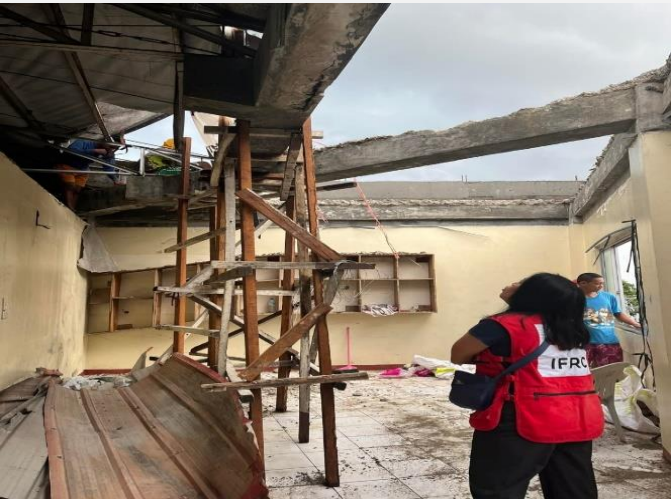
On-going demolition in Bohol Chapter (Photo: PRC)
