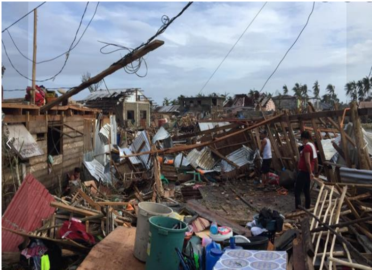
The communities in Surigao Province, Philippines, are left reeling in the aftermath of Typhoon Rai. Homes have been destroyed, infrastructure damaged, and residents displaced. (Photo: PRC)
