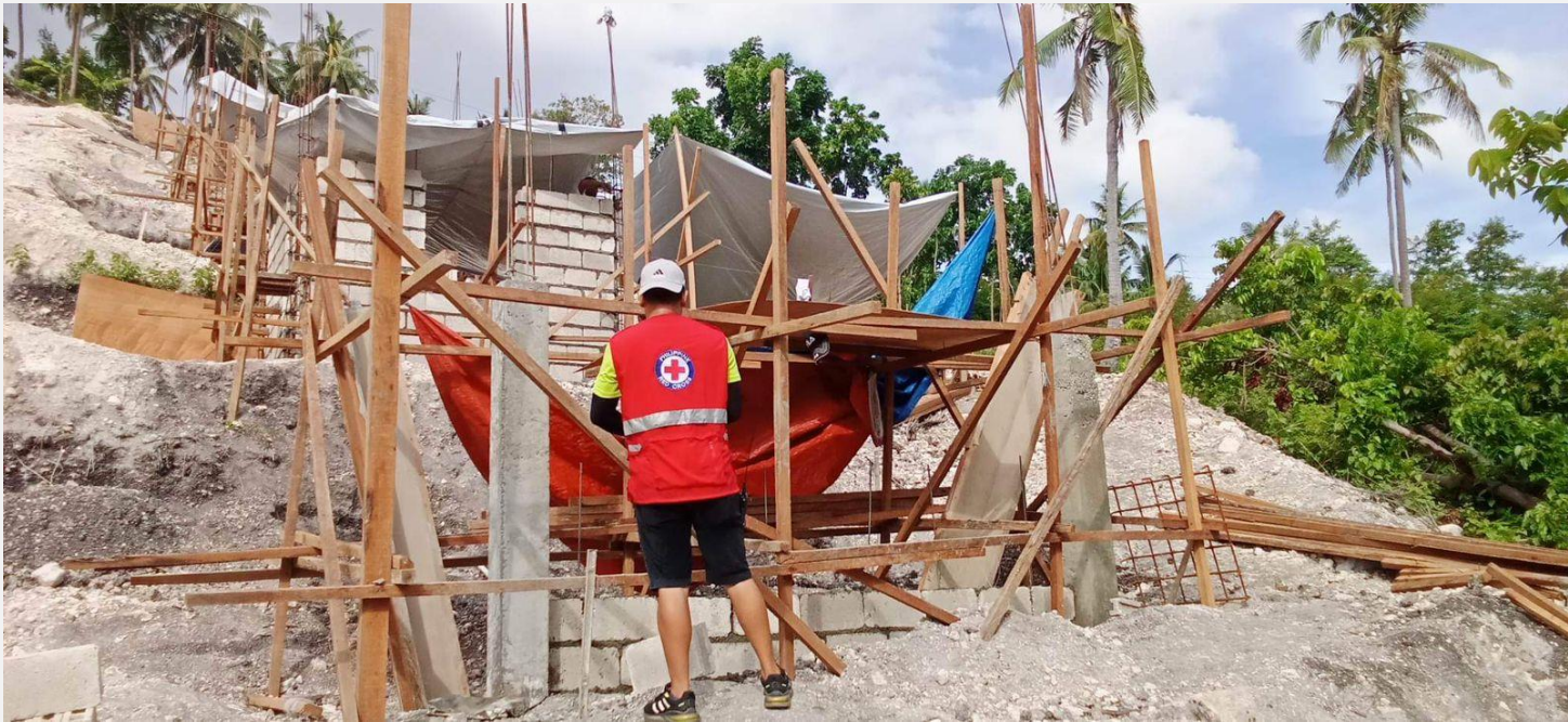
On-going construction of the full shelter assistance program by the Philippine Red Cross in the Municipality of Alegria, Cebu. (Photo: PRC)
