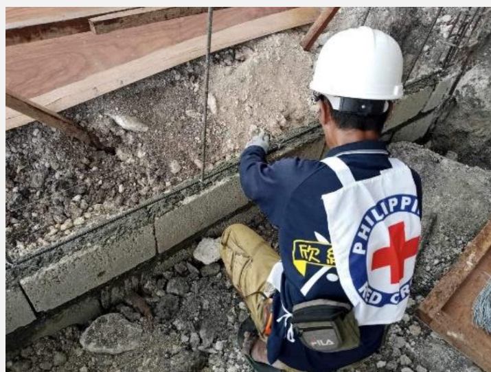
Construction works underway. (Photo: PRC)
