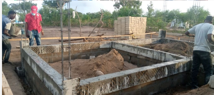
Figure 8: Practical training with master builders
