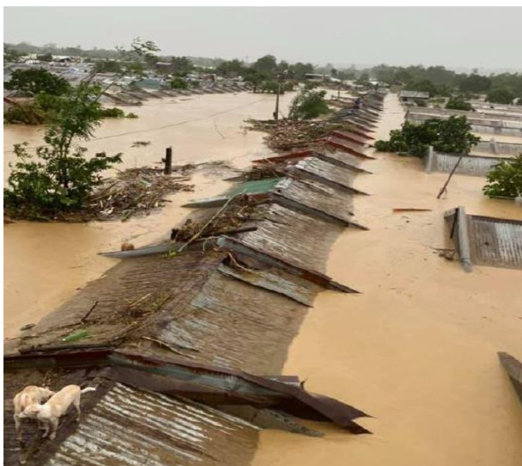
The typhoon caused Flooding up-to roof level (Photo: L Morena)
