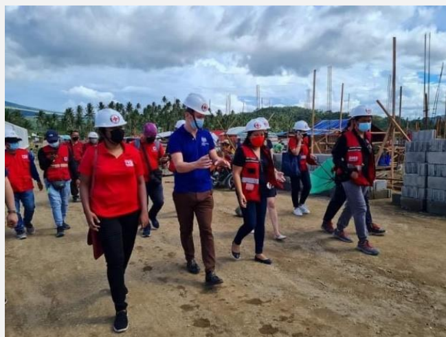
Delegation from the British Embassy in Manila visiting the construction site in Albay together with PRC and IFRC (Photo: PRC)
