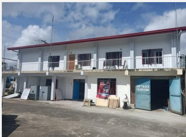
PRC supported the renovation of Catanduanes office. (Photo: PRC)
