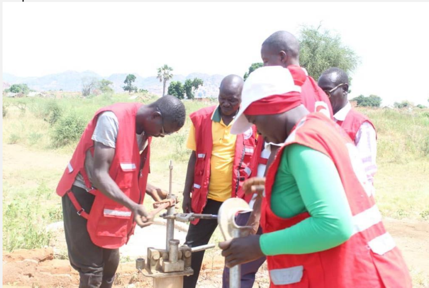
Sudanese Red Crescent Society volunteers repair a borehole. ©SRCS
